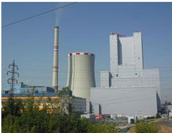
Thermal power station of Ledvice is a part of ČEZ Group. It burns brown coal from the neighbouring Bilina mine and, besides electric energy, it also produces heat it supplies to cities in its surroundings. Older blocks with a total output of 330 MW have been recently supplemented with the most advanced supercritical (600 °C steam) and highly efficient (42.5 %) 660 MW block whose emissions are 20% lower than current technologies.
